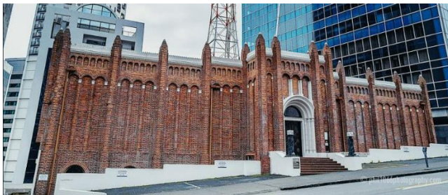
1YA Radio Station Building , 74 Shortland Street, Tāmaki Makaurau/Auckland
