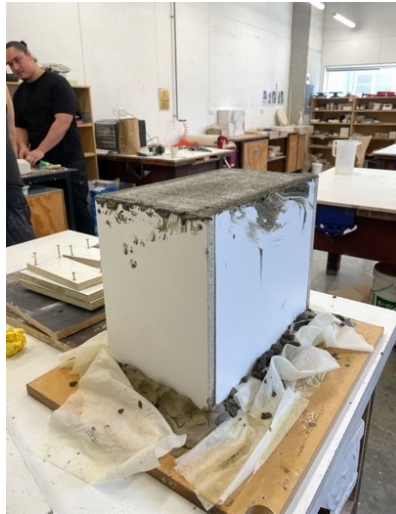
Figure 12. Concrete block construction.
