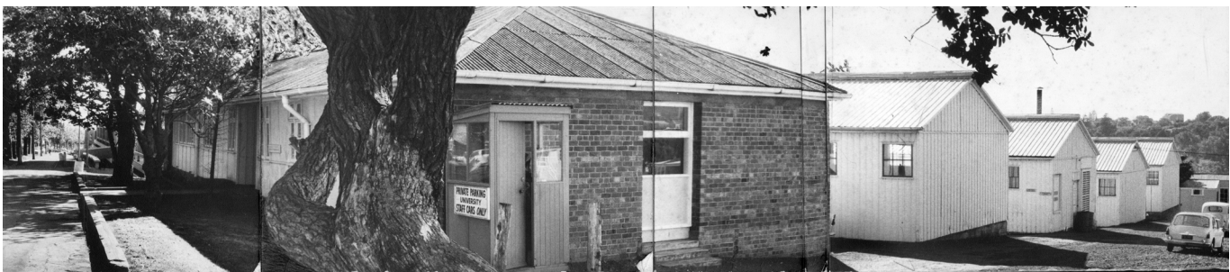
Fig. 2 From the late 1940s, the Auckland School of Architecture occupied old army huts that in the 1970s became the Steel sub-school. [Photographer not known, Architecture Archive, Special Collections, University of Auckland Library and Learning Services, Acc no. 03/10]
