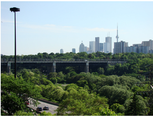
Fig. 1 The Don Valley, one of Toronto's ravines, with Prince Edward Viaduct and the Don Valley Parkway [image from Flickr ( https://www.flickr.com/photos/38693531@N08/4672897942 ), taken by Jess, 2010, Creative Commons licence (CC BY-SA 2.0), no changes made, used here for non-commercial purposes].
