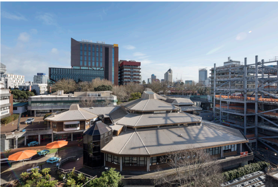
Fig. 1 The complex roof forms, with the Architecture and Planning Library in the foreground. It sits back-to-back with the Design Theatre (under the turret), with the Dean's Office to its left (south), and the Conference Centre Lecture Theatre and so-called Flat Floor Space to the right (north). Construction of a new building for the Faculty of Engineering is underway.
