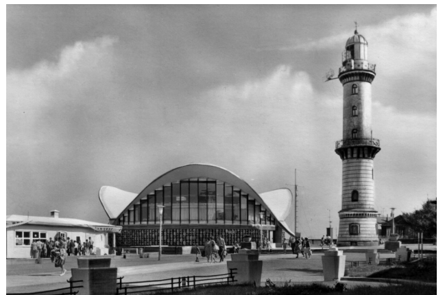
The Teapot (Teapot) restaurant in Warnemünde (1968). Shell structure consisting of three hypar shells, thickness 7cm, radius 20m
