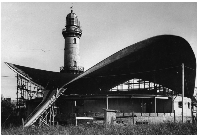
The Teapot (Teapot) restaurant in Warnemünde (1968). Shell structure consisting of three hypar shells, thickness 7cm, radius 20m
