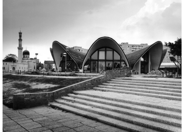
The Seerose (Water Lily) waterfront pavilion in Potsdam (1983). Eight-part rosette made from hyperboloid shell segments, thickness 7cm, diameter 23m.
