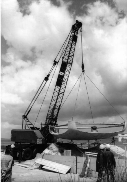
Strandwache 2 (Lifeguard 2) in Binz (1981). Two double-curved shells assembled to form a box, thickness 3-5cm, 5.5x5.5m
