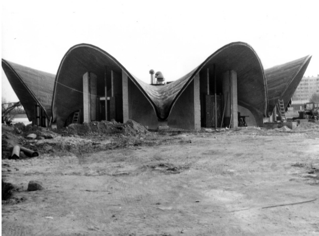
The Seerose (Water Lily) waterfront pavilion in Potsdam (1983). Eight-part rosette made from hyperboloid shell segments, thickness 7cm, diameter 23m.
