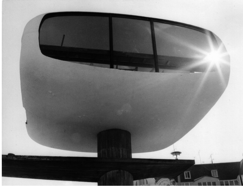
Strandwache 2 (Lifeguard 2) in Binz (1981). Two double-curved shells assembled to form a box, thickness 3-5cm, 5.5x5.5m
