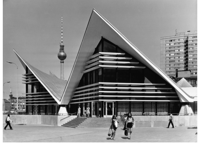
The Ahornblatt (Maple Leaf) restaurant in Berlin (1973). Five assembled hyperboloid shell segments, thickness 7cm, 5x22x35m
