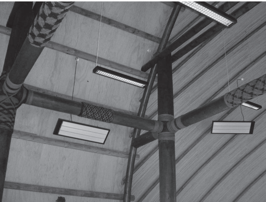
Figure 3: The lashed joint as an occasional feature
