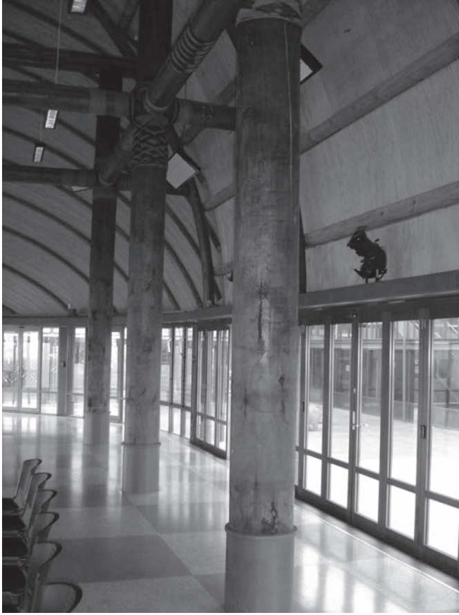
Figure 4: The interior poutu (posts) structure the space
