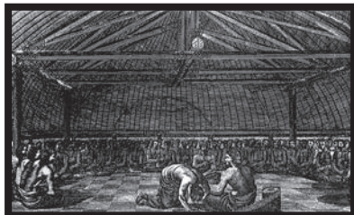
Figure 1: Inside the Falehau, Tonga, in 'A new, authentic and complete collection of voyages round the world ...' London 1784. The image shows the tectonics with lavalava connecting the structure.
