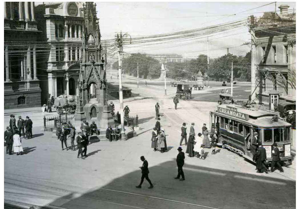
FIGURE 6. Custom House Square Underground Comfort Station, 1919, DCC Archives
